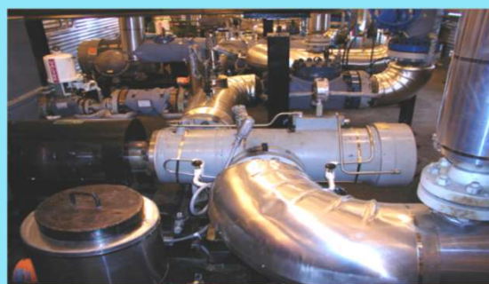
Crude oil booster pump L3HG-xxx 50 m 3 /h @ 103 bar
