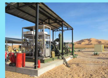
Multiphase Pump L4MG-200 517 m 3 /h @ 17.5 bar
