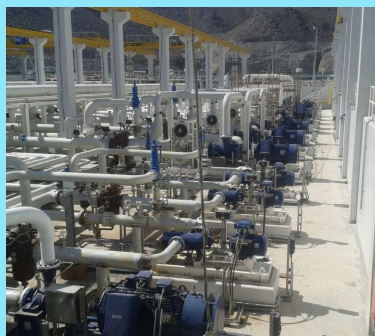
Fuel Oil transfer pump L4MG-220 1,530 m 3 /h @ 12 bar
