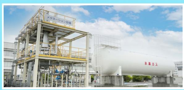
Methanation is a technology for synthesizing e-methane from hydrogen and  $CO_2$ . It is required to develop efficient, large-scale methanation facilities to replace conventional natural gas with e-methane.
