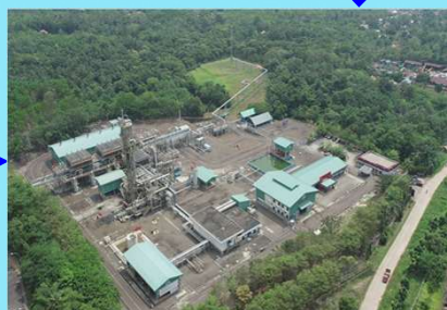
Extraction Plant Prabumulih
